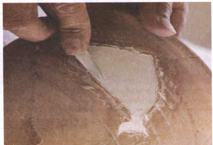
Figure 13: excess plaster is cut away with a scalpel or other tool
